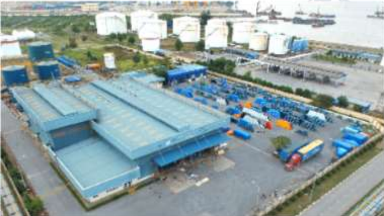
CHEVRON LUBRICANT PLANT
