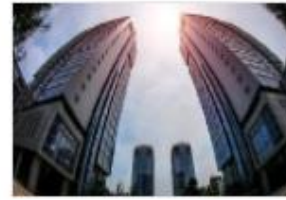
Chongqing Internet Industrial Park
